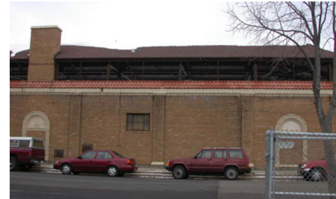
FIGURE 21: Southwest grandstand façade. (2002)
