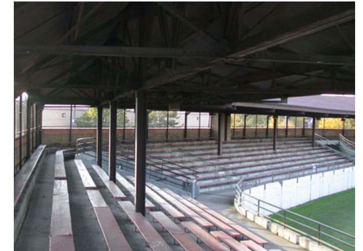
FIGURE 22: Section B bleacher section looking northwest. (2002)
