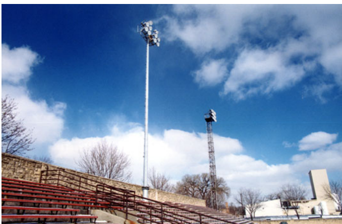
FIGURE 70: Two different styles of field lighting towers. (2002)
