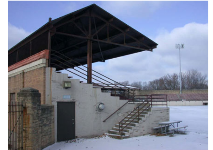
FIGURE 15: East end of Section A grandstand. (2002)
