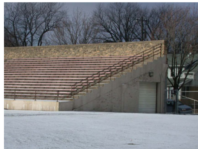
FIGURE 47: Northeast end of the section E bleachers. (2002)
