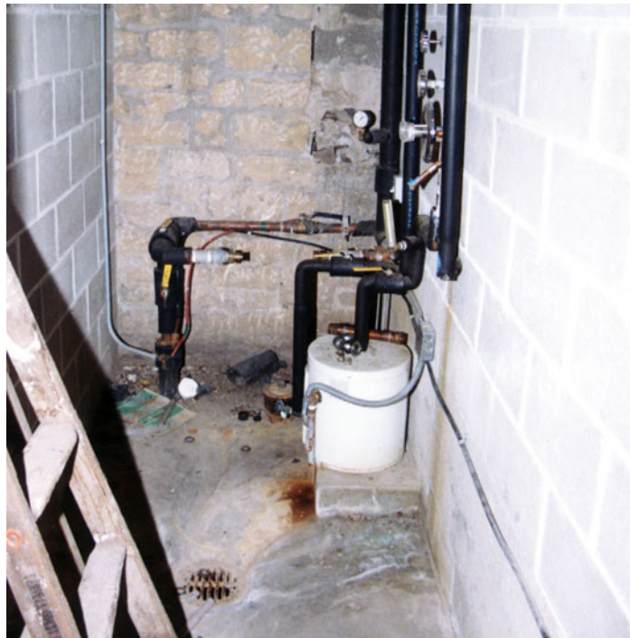
FIGURE 56: Newer copper piping tied into original steel pipes. (2002)
