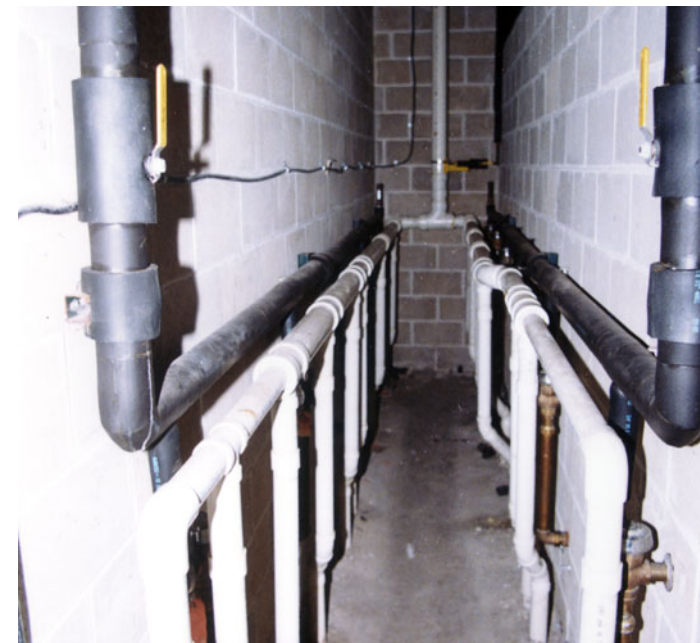
FIGURE 57: New PVC sanitary drainage piping. (2002)
