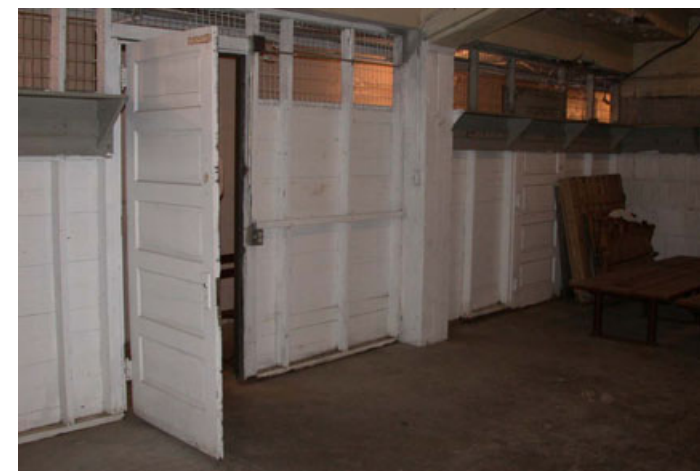
FIGURE 25: Locker room looking toward the corridor. (2002)
