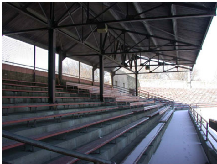
FIGURE 31: Section C grandstand looking north. (2002)
