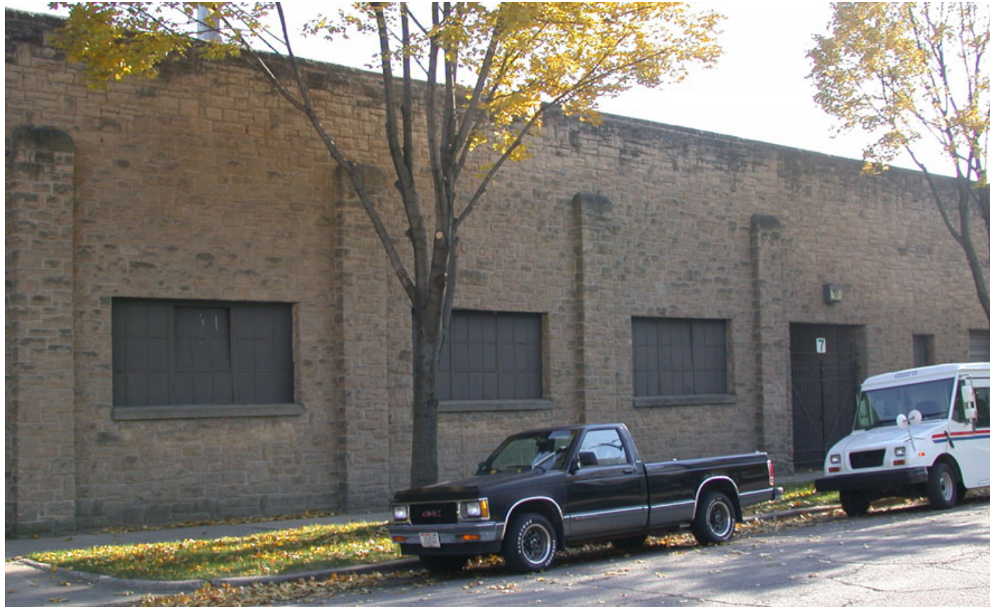
FIGURE 44: North end of the northwest façade. (2002)
