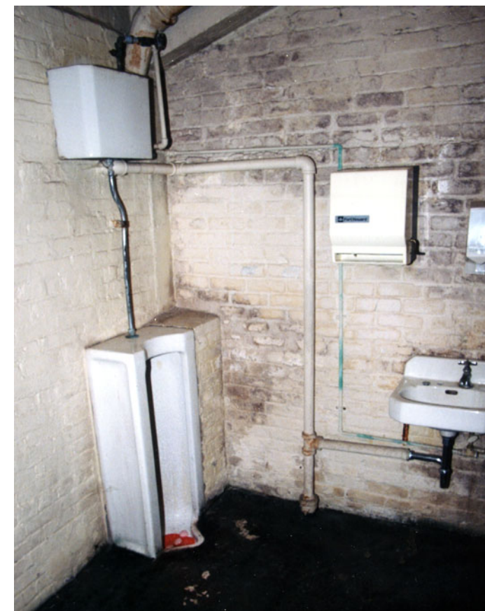
FIGURE 58: Toilet room with original cast iron and steel piping. (2002)
