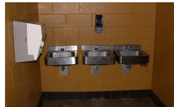
FIGURE 42: Lavatories in the Men's rest room. (2002)
