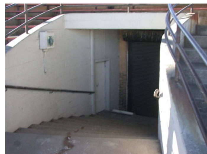
FIGURE 32: Pedestrian entrance with roll down door. (2002)
