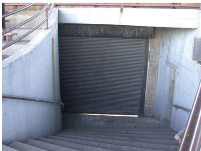
FIGURE 16: Pedestrian grandstand entrance with roll down door. (2002)
