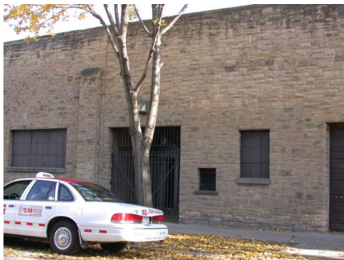
FIGURE 46: Gate 7 entrance and ticket booth. (2002)
