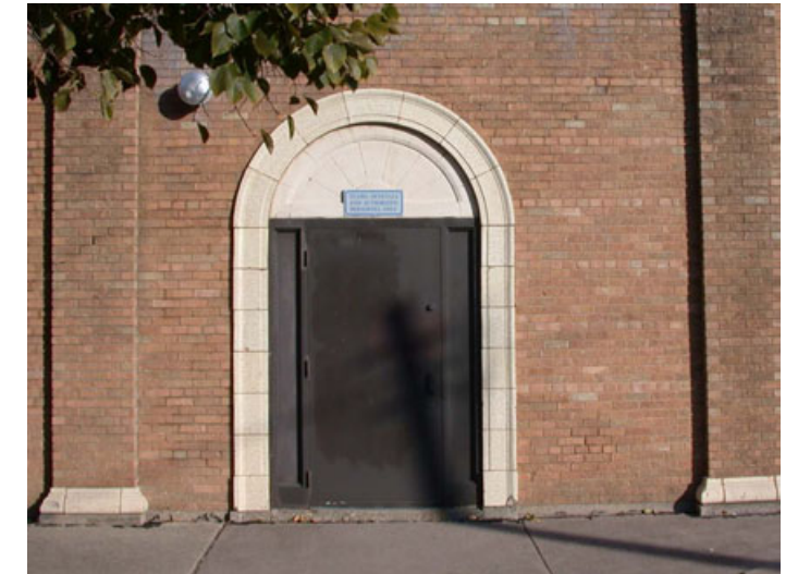
FIGURE 8: Modern entrance door, sidelight and frame. (2002)
