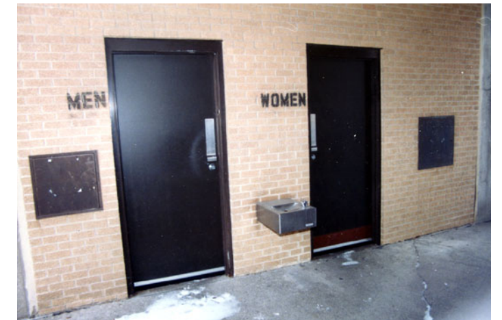
FIGURE 59: Vandal-resistant stainless steel fixture. (2002)
