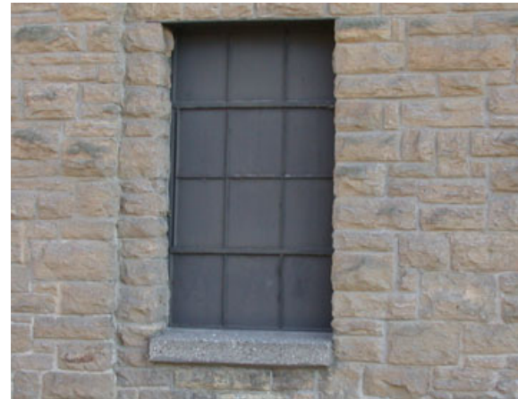
FIGURE 5: Typical steel window. (2002)
