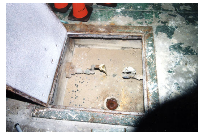
FIGURE 55: Former location of the water meter. (2002)
