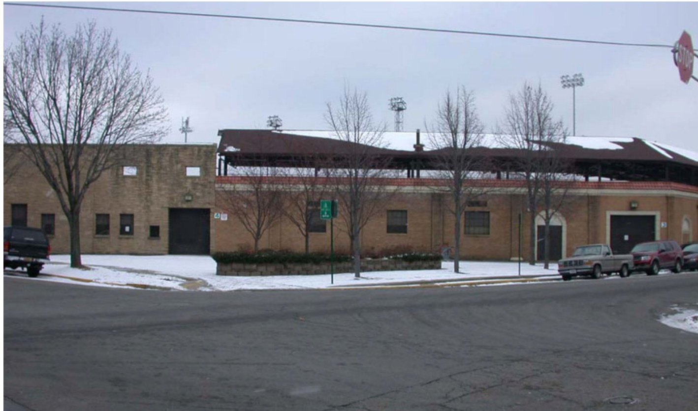
FIGURE 28: West façade of original and 1934 grandstand sections. (2002)
