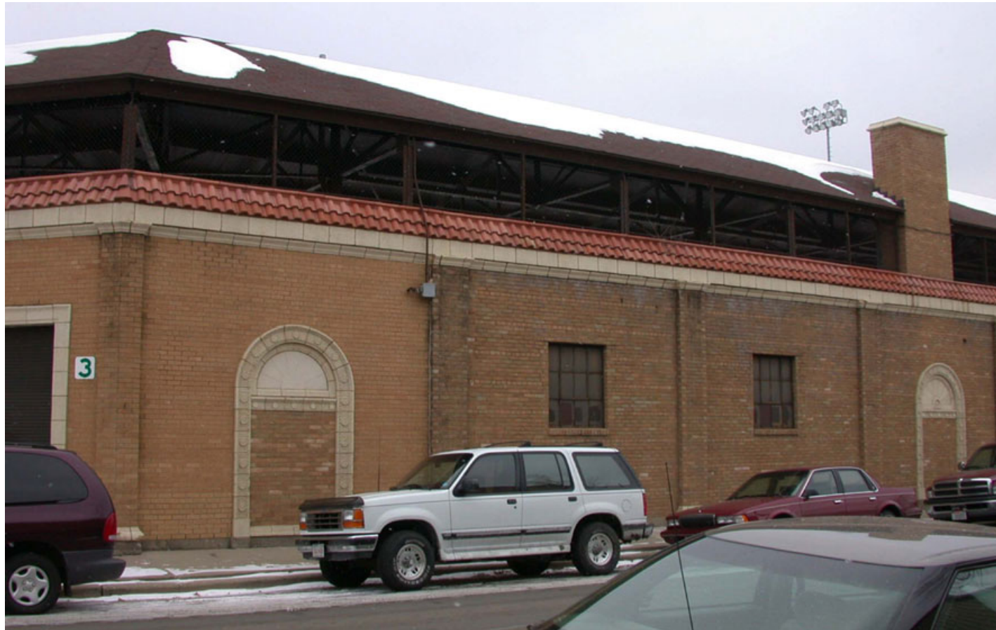
FIGURE 20: Southwest grandstand façade. (2002)
