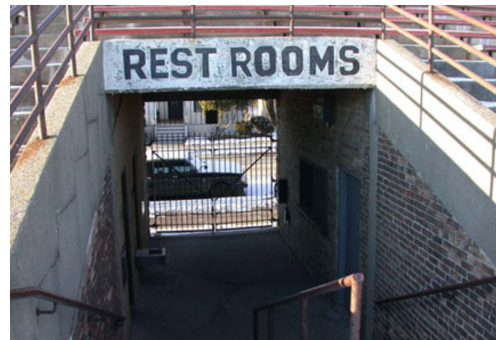
FIGURE 38: Stair leading to the public rest rooms. (2002)
