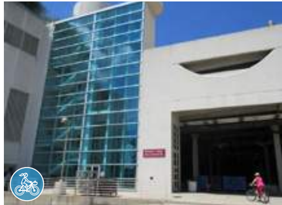
Figure B.12 Monona Terrace Bike Elevator
