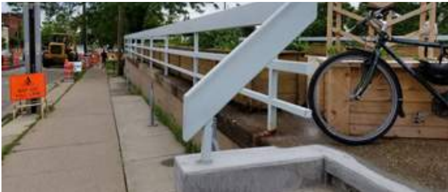
Figure B.16 MWU Water Reservoir Building Interfacing with East Wilson St Sidewalk
