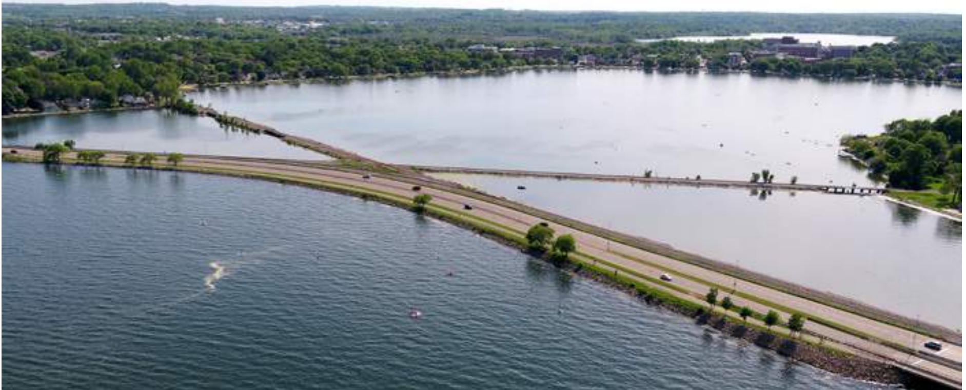
Figure 4 John Nolen Drive Causeway View Looking Southwest
